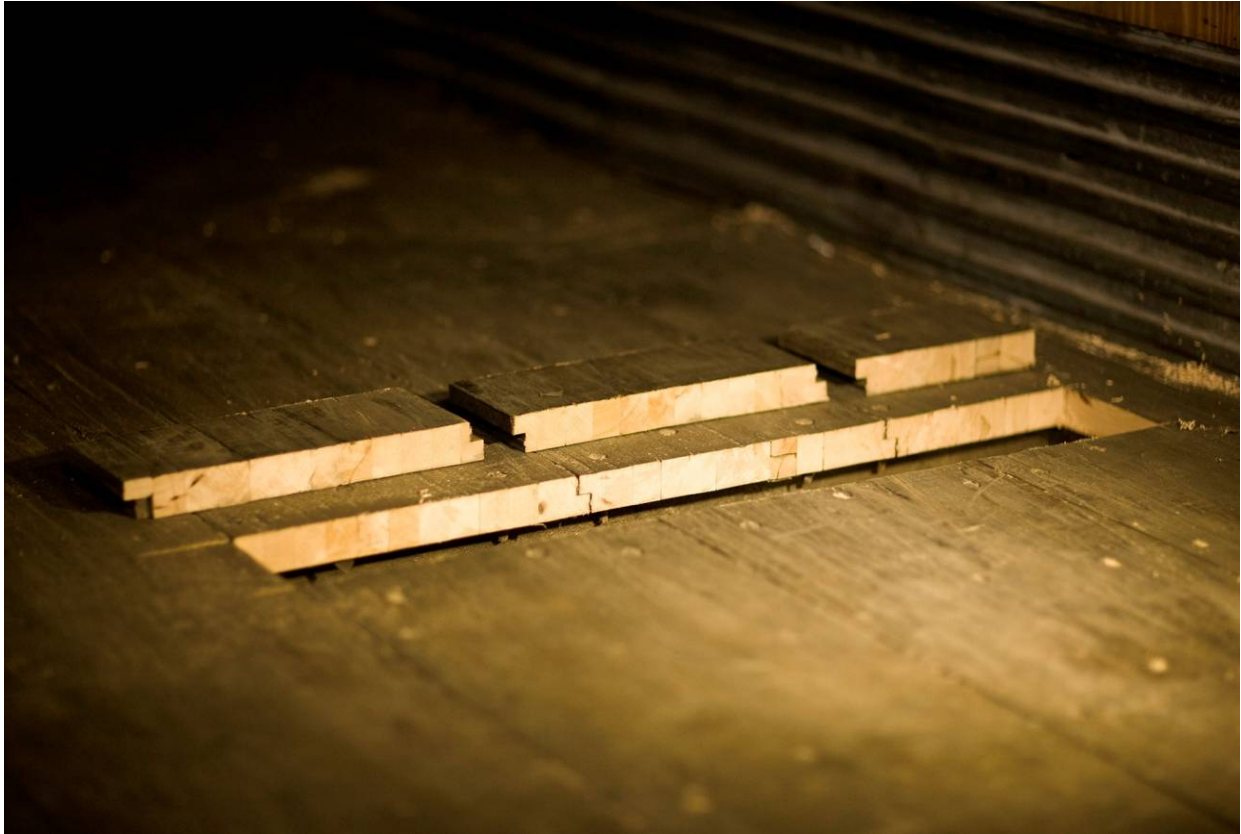
Figure 59. Photograph. Wooden floor cut section.
